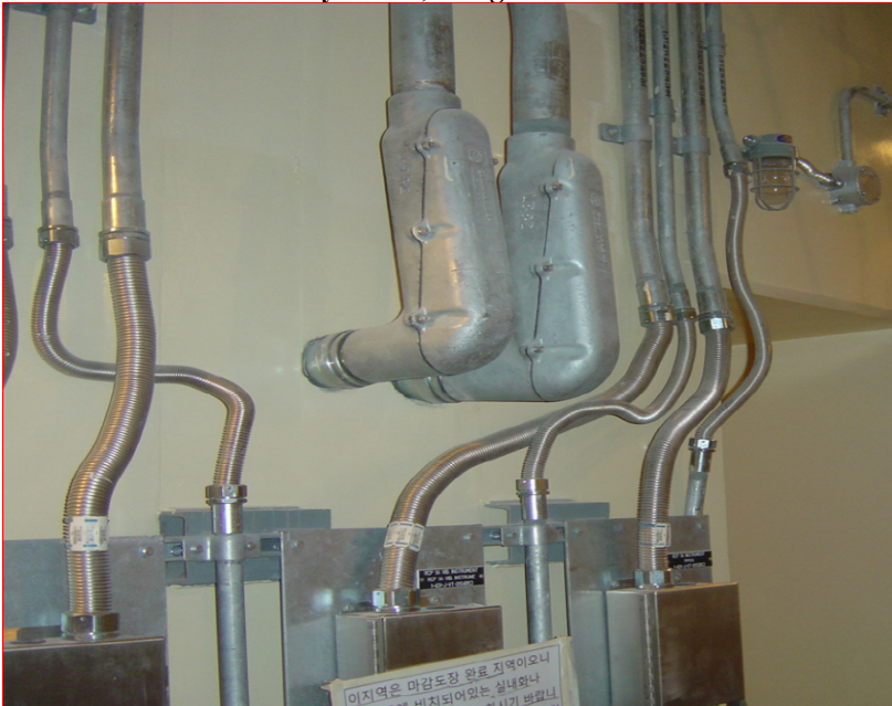
Figure 6.11.1. Example of interface between cable trays and conduits. Flexible conduits shall be used for Instrumentation and safety cables, being the aerial connection for non-safety power cables.
