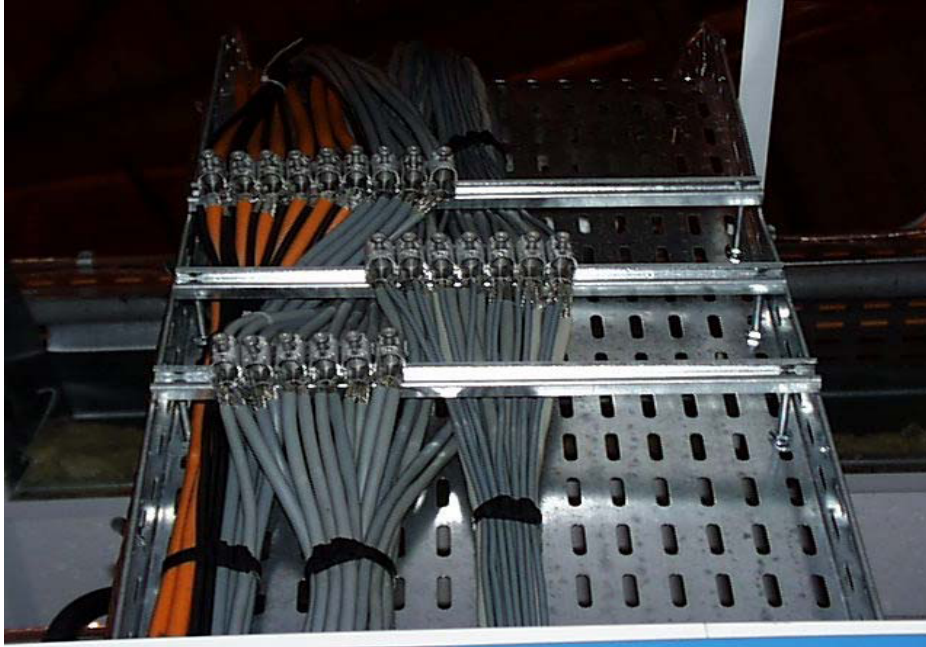
Figure 9.4 Spring clips installed on cables
