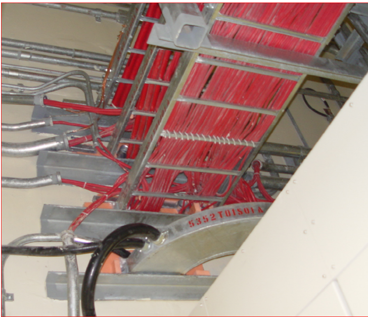
Figure 6.11.1. Example of interface between cable trays and conduits. Flexible conduits shall be used for Instrumentation and safety cables, being the aerial connection for non-safety power cables.
