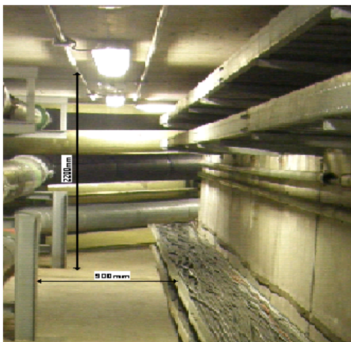
Figure 5.7.4 Technical gallery between experiment hall and service building
